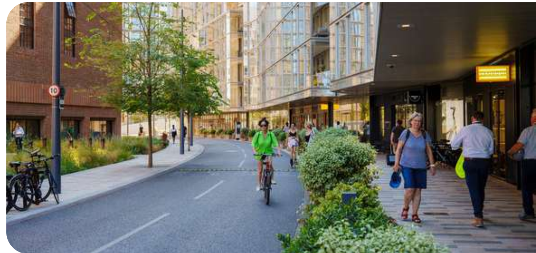
Shared carriageway, with low design speeds and traffic volume, suitable for cycling and wheeling, Battersea, London.
