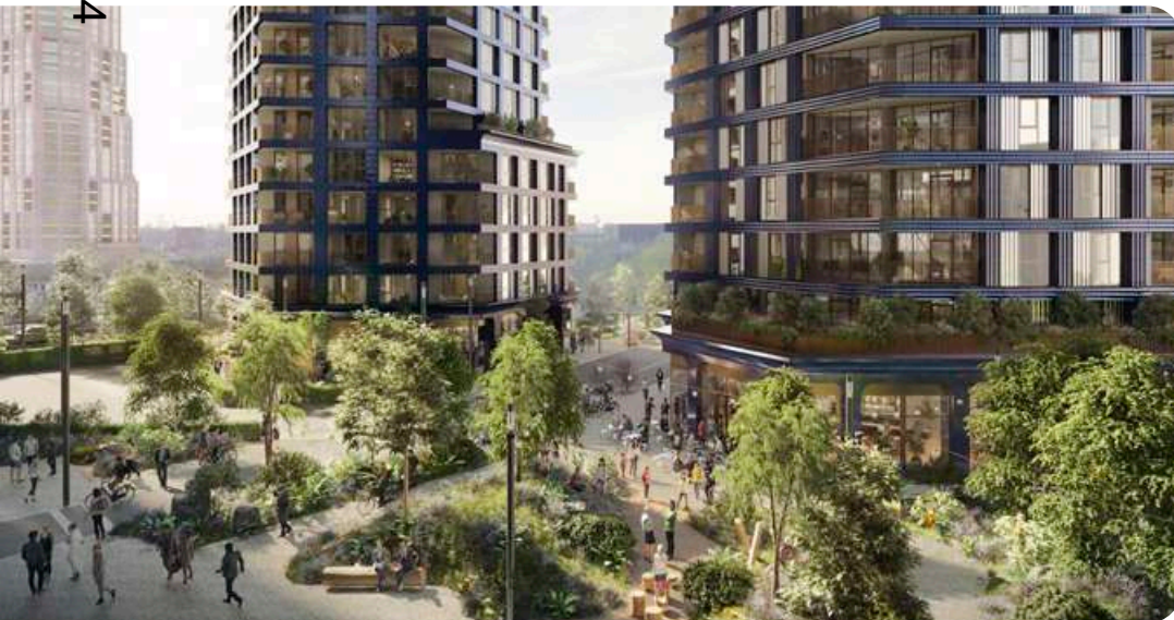
High-density development achieving UGF through green roofs and predominantly green open spaces, International Quarter London
