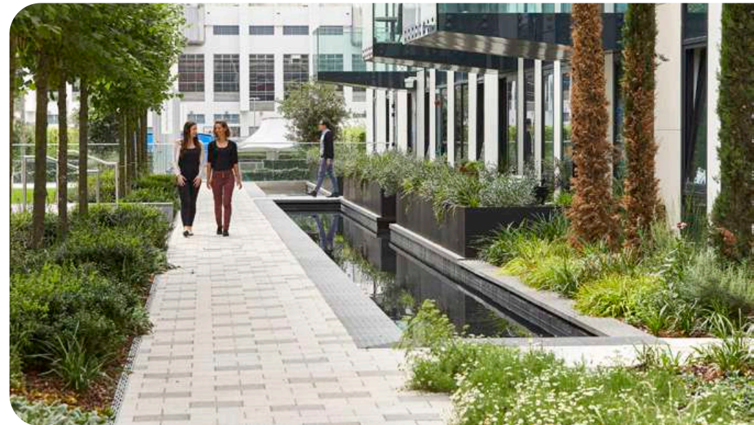
High quality communal space for residents incorporating planting, seating and water features, Wembley, London.
