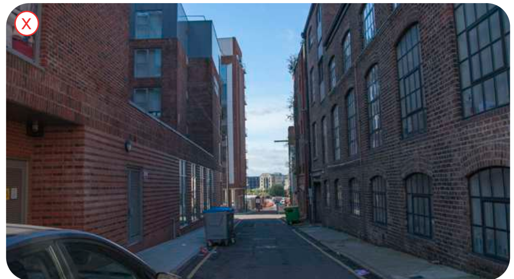
A high street height to width ratio, of more than 1:1, results in poor daylight access and privacy issues, Liverpool.
